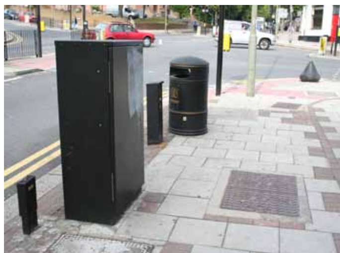
Reduce street clutter - Regents Park Road
