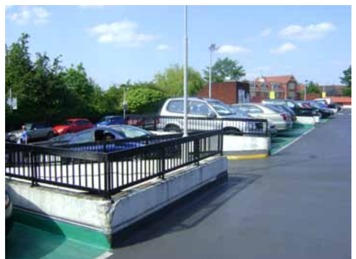
Tesco multi-storey car park
