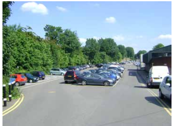
Finchley Central car park
