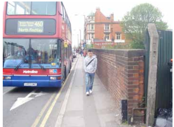
The bridge over the railway lines
